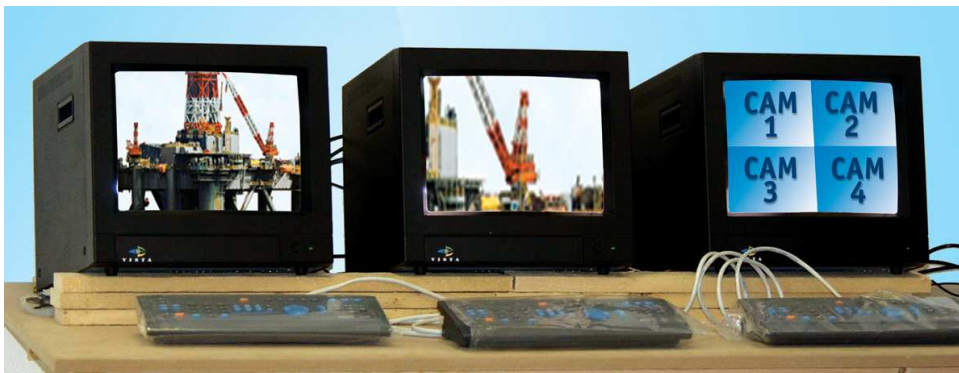
Typical Safe Area CRTs and Consoles
